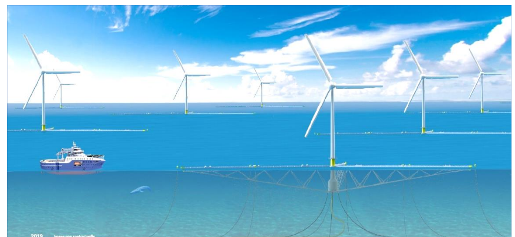
Figure 12 - two examples of HACE module integration with marine infrastructure for asset protection and energy provision. Above, a marina with modules integrated into the boundary. Below, floating wind turbines with modules integrated into their bases. The combined wind-wave device can use a single cable for electricity export.
